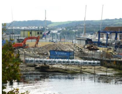
October 2013 Demolition complete
