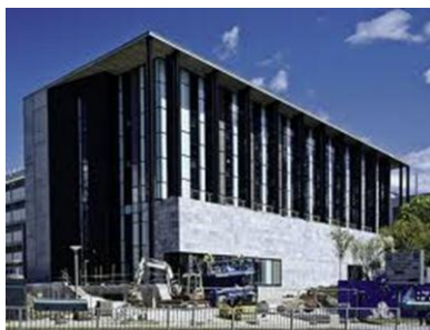
The new marine building at Plymouth nears completion.
