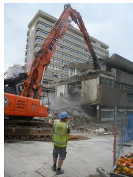
The demolition of the Isaac Foot Building, built in 1962, as the Cadets Dining Room commences.
